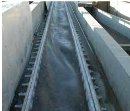
Fluachem Elastomer installed in a horizontal duct.
