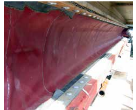
Fluachem Fluoropolymer installed in a vertical duct.
