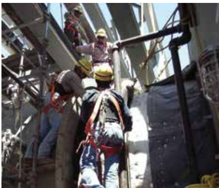
Fabric expansion joint installed over the manifold.
