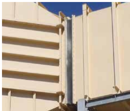
Acouseal installed in gas turbine air inlet.
