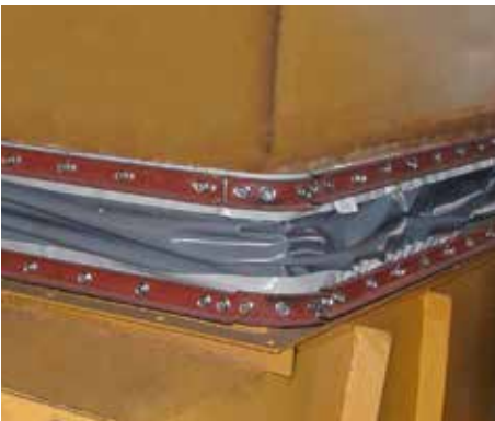
KE-Flex installed in an air duct.
